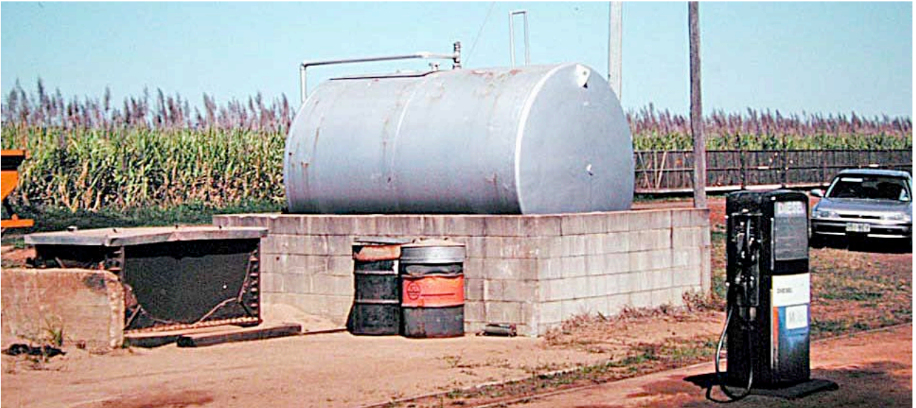
The loco fuel bowser and storage tank with spill containment barrier in 2000. The bowser can be seen in the middle distance through the open shed in the previous photo. Greg Stephenson photo from the CaneSIG collection.
