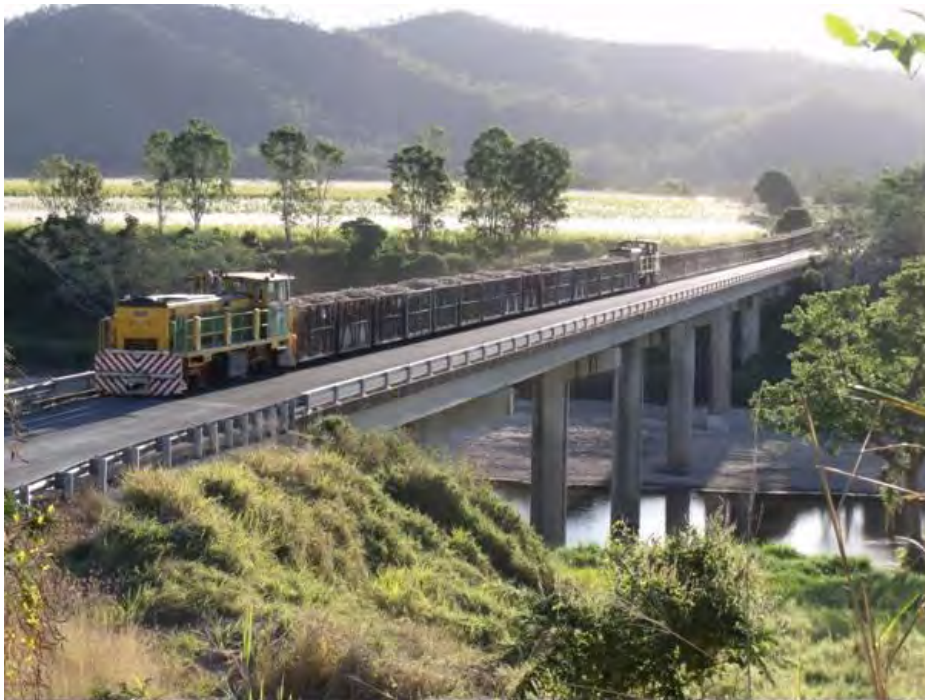
The “John Luscombe Bridge” remains in use as part of the Mackay Sugar Cane Railway Network.
