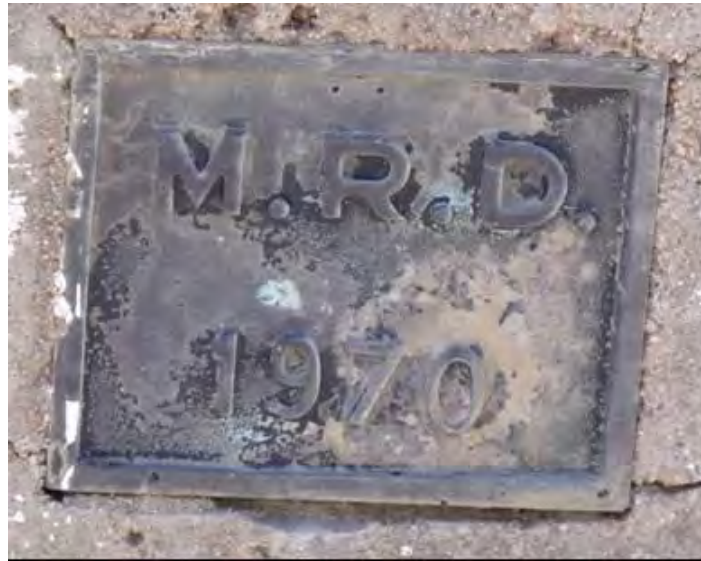
Date Plate cast into the replacement bridge.
