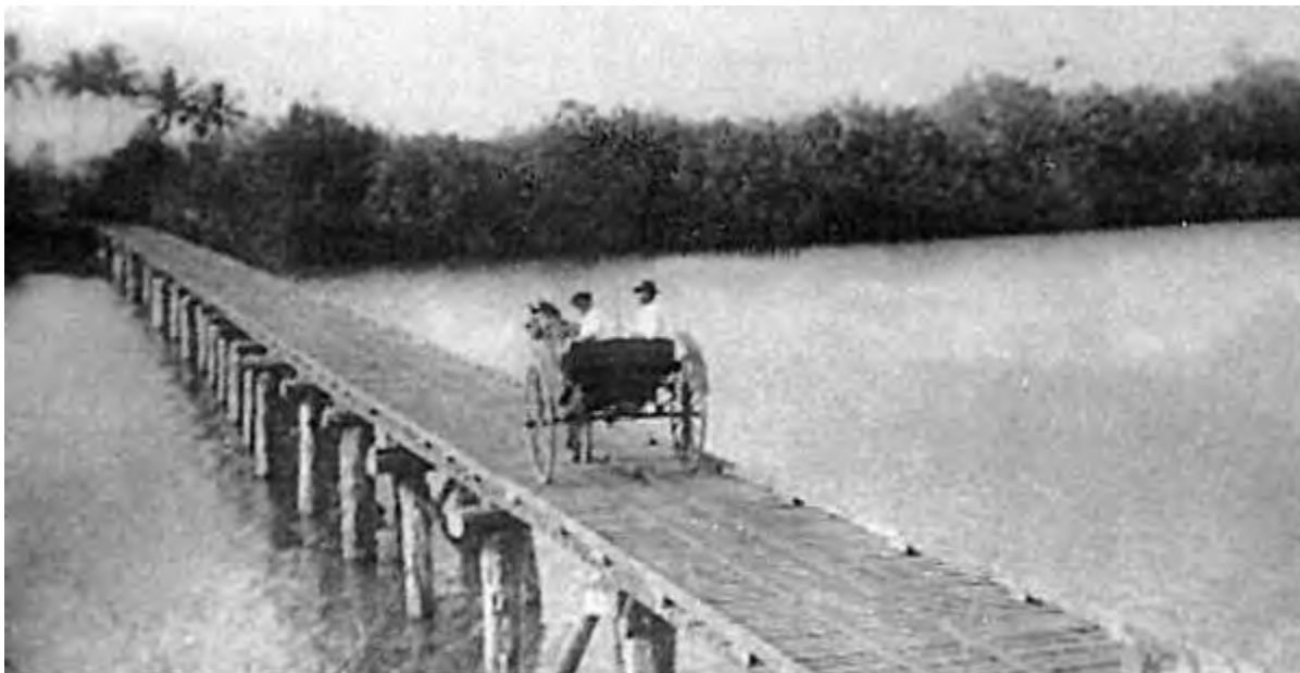
Original Barron River bridge, Stratford. Image: Cairns Historical Society (B3669).
