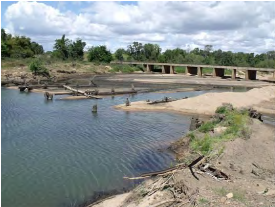
In the background, the cane railway bridge is in front of the road bridge. In the foreground are the remnants of the original timber bridge.
