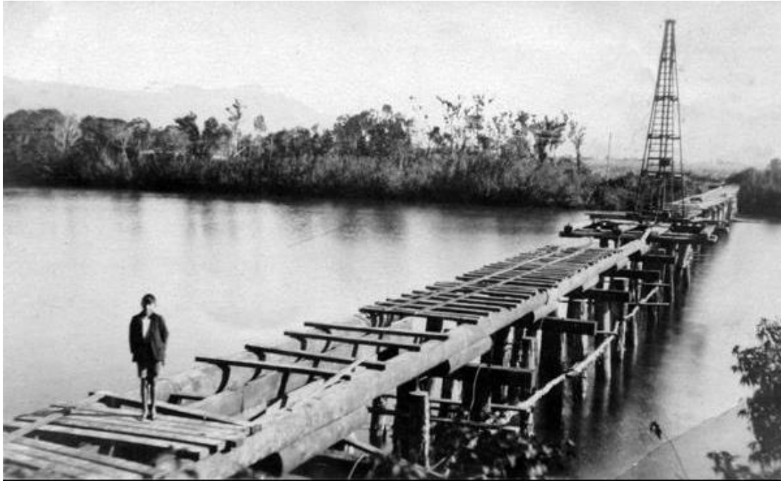
Farmers' Bridge being repaired, 1927. Image: Les Humphries.
