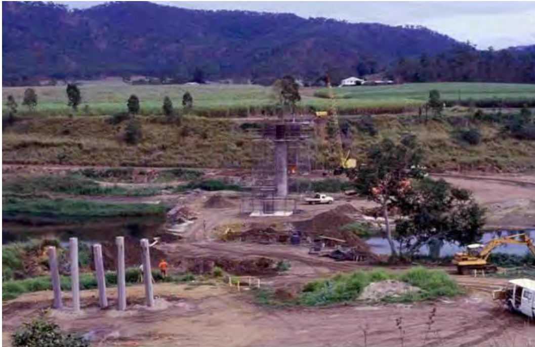
Construction of concrete piled foundations and piers in 1986.
