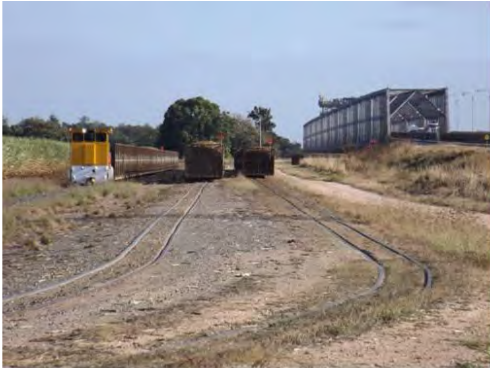
Dual purpose Road/Railway Bridge over Burdekin River Bridge, Home Hill
