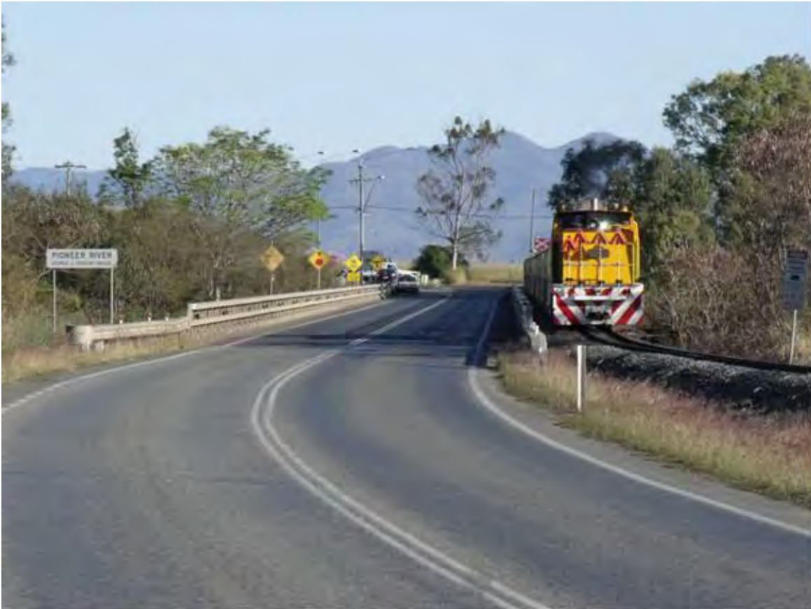
The bridge shares common piers and abutment to the top of the headstocks. The road and tramway are separated on the superstructure.
