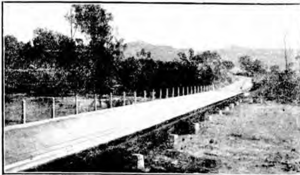
The bridge over the Houghton River (built by the Main Roads Commission) on the road leading to the sugar mill at Gira south of Townsville. It is constructed of timber, with concrete piers. It is a dual purpose bridge—designed to carry ordinary traffic and also steam tram traffic from the canefields. One of the features of this bridge is that it has a concrete coping.
