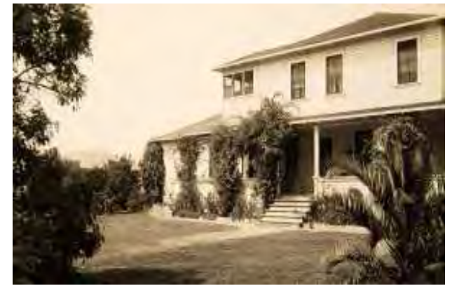
#5. The Club House at Betteravia was quite a grand building. Again, the palm tree attests to the passage of time!
