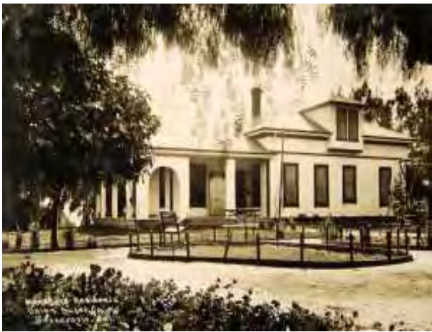
#1. This is the site of the Plant Managers large impressive house. The terrain drops off just behind where the house stood, to a large depression that once contained a natural lake.
