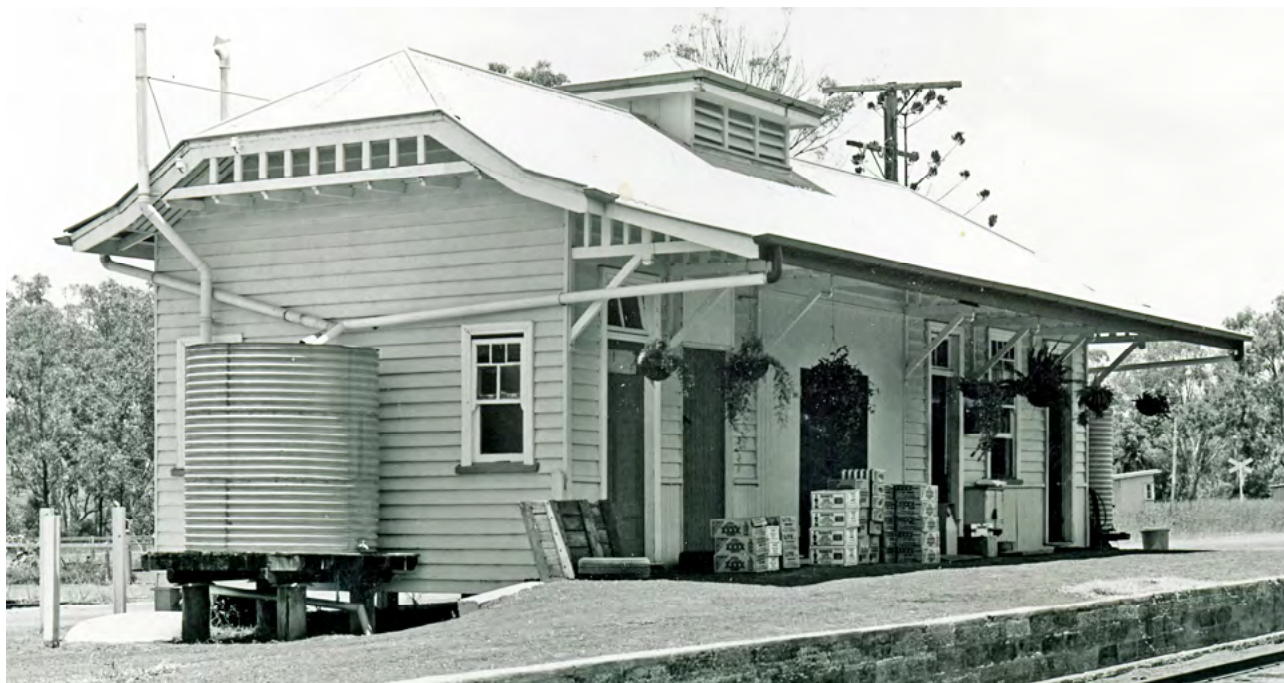
Yarraman station still looked like a railway building when photographed in 1989, a few months after it had seen its last train. Most of Yarraman's yard infrastructure was still in place at this time (and the hanging baskets were still being tended) although the building was by then being used as a road freight depot. At some stage during or after the 1960's the passenger waiting area had been enclosed, presumably to provide additional storage space.
