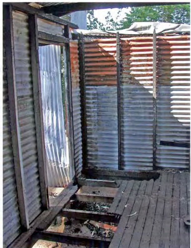
BELOW: Interior view towards the back door showing some of the vandalism. Note the very simple framing for both wall and door.
