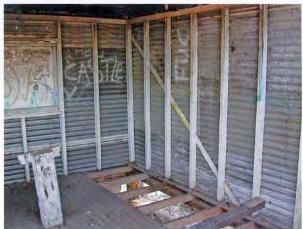
BELOW: Interior view towards the back door showing some of the vandalism. Note the very simple framing for both wall and door.
