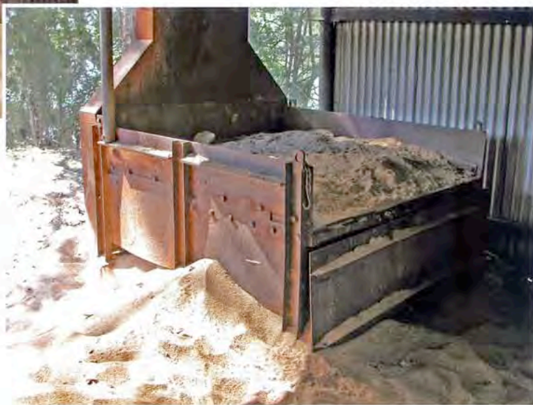
ABOVE: Back side of the sand drying shed showing the dryer, dryer chimney, shed roof framing and interior construction. Note the construction-style adjustable steel post holding up the roof joist.
