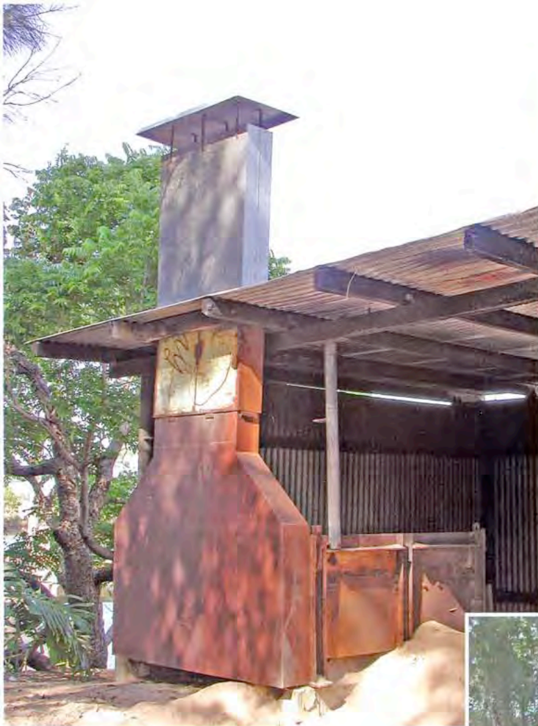
ABOVE: Back side of the sand drying shed showing the dryer, dryer chimney, shed roof framing and interior construction. Note the construction-style adjustable steel post holding up the roof joist.
