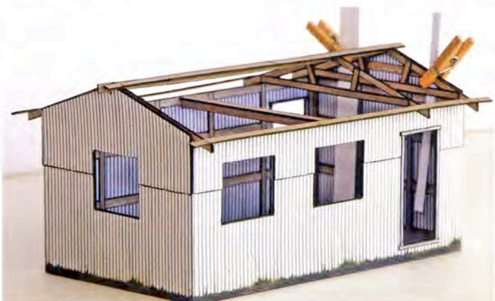
ABOVE: Lunch room walls assembled with floor in place and 't-bar' fitted to keep the side walls from bowing in. Roof construction begun with one truss fitted at the close end and two at the other. The ridge board and three purlins currently hold the trusses in place, an additional seven purlins, as well as wind blocks, will complete the framework for the removable roof. The card spacer strips visible at the far end ensure that the roof module is removable
