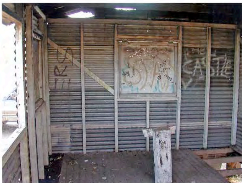
BELOW: Inside view of the end and front wall showing the framing and the window cover, hinged at the top for opening. The front wall and other end do not have the cyclone cross-bracing.
