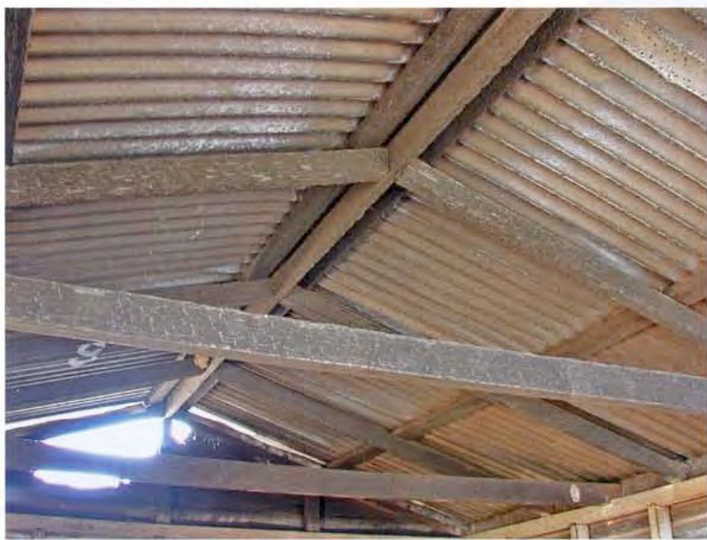
BELOW: Inside view of the end and front wall showing the framing and the window cover, hinged at the top for opening. The front wall and other end do not have the cyclone cross-bracing.
