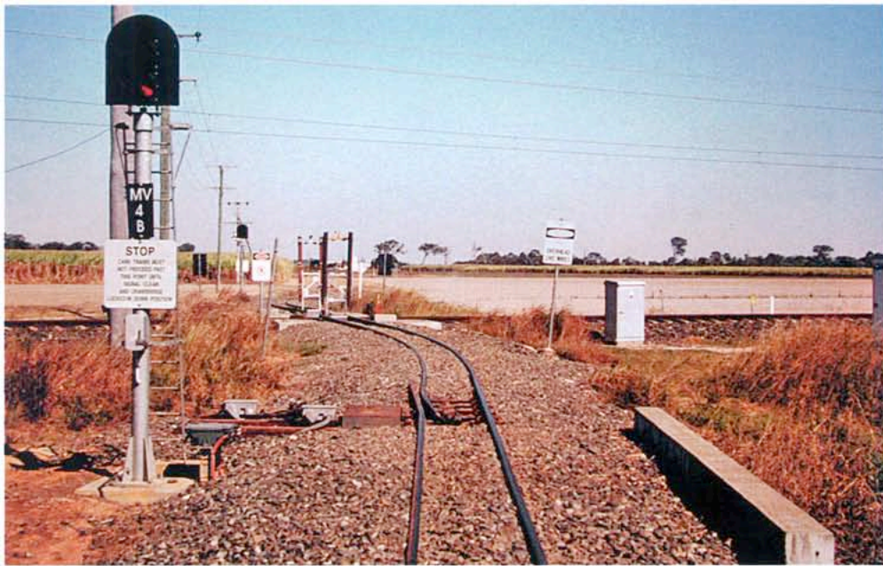
LEFT: Signals and check rail on the approach to the Pleystowe Mill's drawbridge over the QR line at Wollingford, 1995. The sign to left reads 'STOP, Cane trains must not proceed past this point until signal clear and drawbridge locked in down position'. The centre sign is the 'Keep Clear' sign detailed in the other photo, and the sign on the right is a standard QR warning about overhead live wires. Greg Stephenson photographer.
