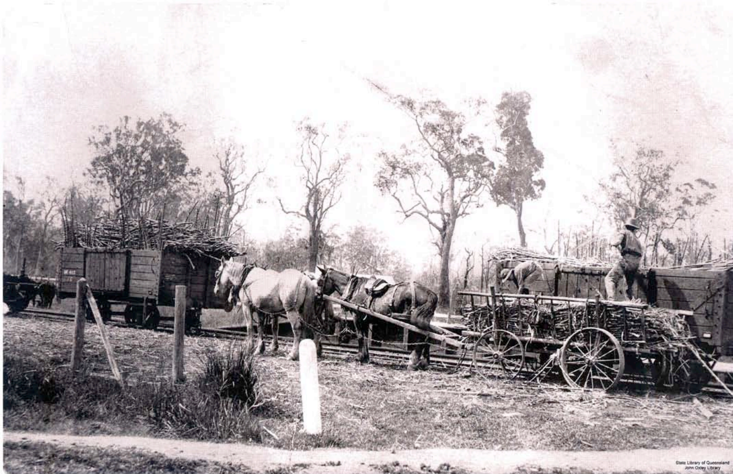
ABOVE: Manually loading wholestick sugar cane into Queensland Rail four wheel DF (firewood) class wagons at Pomona, around 1910. The cane in the front wagon (DF 412) is loaded above the sides and has a rough fence of upright stalks holding the load in place. In other areas the cane stalks were stacked upright in the wagons. State Library of Queensland image.
