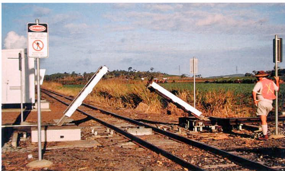
LEFT: Lowering the Pleystowe Mill drawbridge at Wollingford, 1995. The 'Danger' sign reads 'Keep Clear, Bridge Operates Automatically, Authorised Access Only'. Greg Stephenson photographer.
