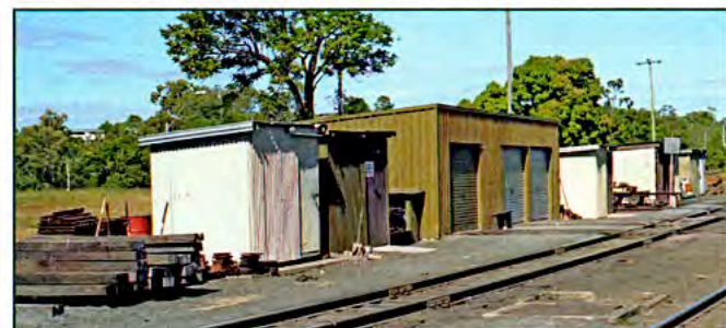
BELOW: A modern colourbond sheathed navy shed with roller doors (centre) for use by section cars, road/rail and other navy vehicles in QR's Sarina maintenance precinct, 1990. Given its age, it's likely that the shed has a concrete floor. The older four stall shed is two buildings beyond.
