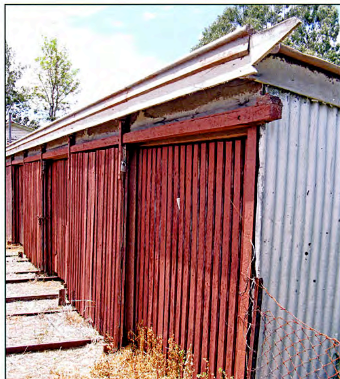
ABOVE: This is the reference photo used to create the texture for one of the doors and to scale the size of the shed. The door is 6' 4" wide and it is 8' 0" from the ground to the top of the roof, all other dimensions have been scaled from these two measurements. The model's roof has more overhang than this shed, but the overhang dimension seems to have been flexible, perhaps depending on when the shed was built.
