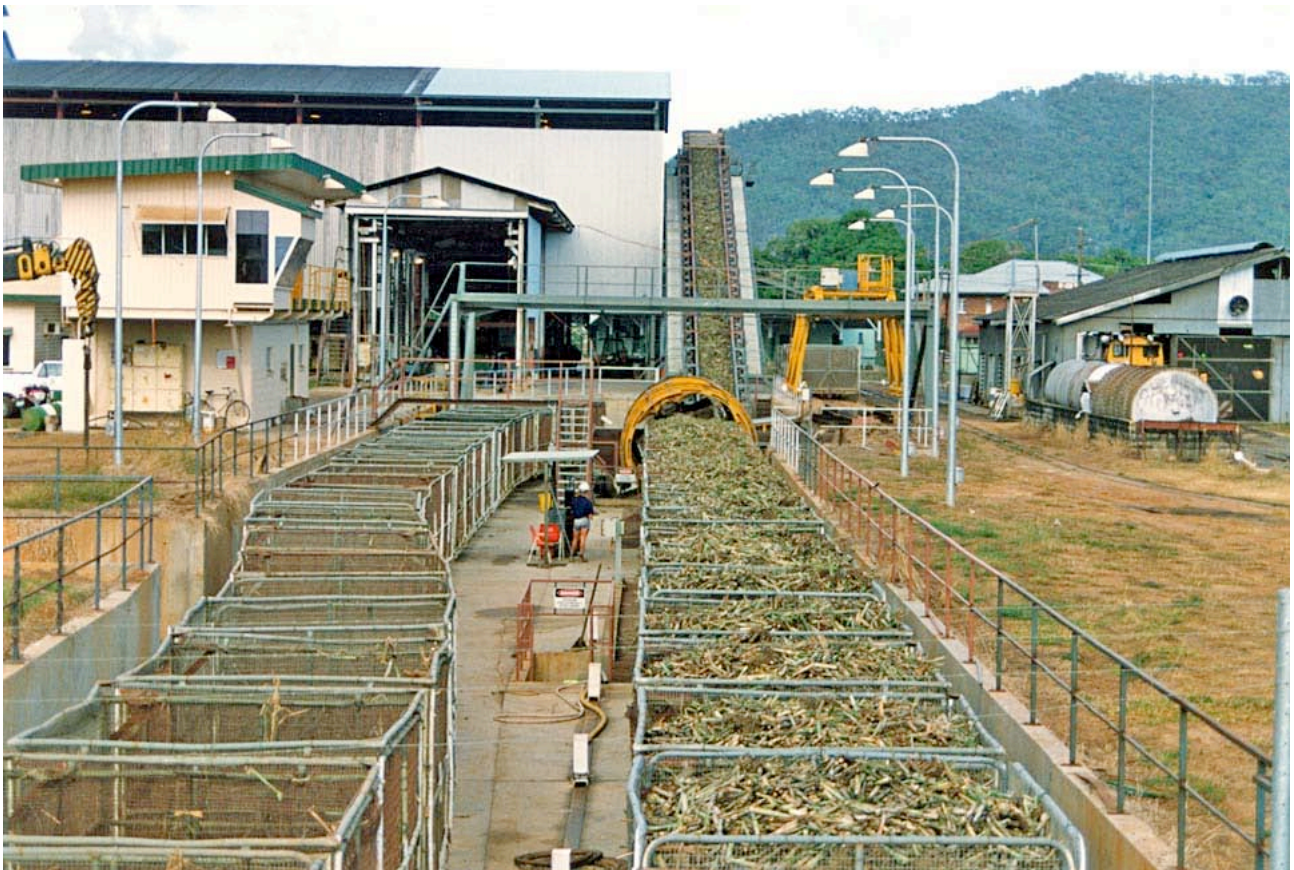
Empty and full lines run side by side on the dead end layout of Gordonvale's Mulgrave Mill
