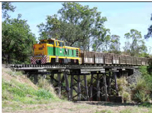
Mackay Sugar – Palm Tree Creek, Garbutt Former Netherdale Branch. Typical QGR timber trestle bridge is now used by cane trains.
