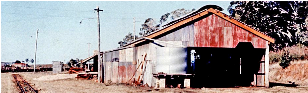
Huxley depot of Isis Mill, note the cutout section to accommodate a taller steam loco. David Mewes photo, 1969.
