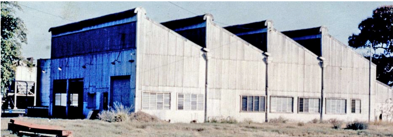
The old shed at Kalamia, a typical saw-tooth roof industrial building. David Mewes photo, 1975.
