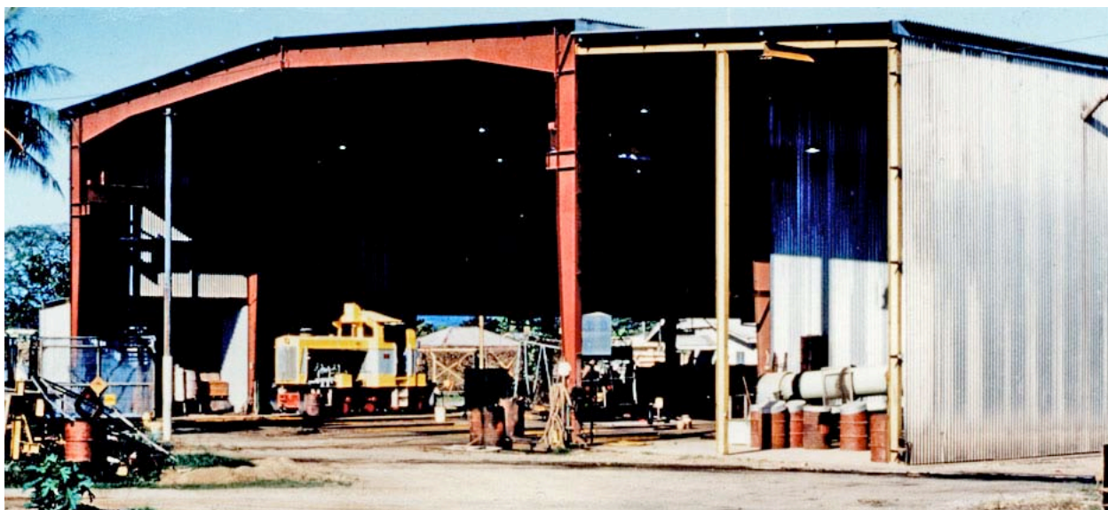
New shed at Mourilyan, a tall and spacious portal framed extension of the mill building. David Mewes photo, 1984.
