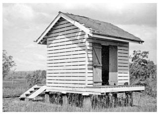
Nurinda on the Brisbane Valley branch, exemplified the typical standard cream shed, but it was also one of the less common structures to feature a 'fibro' slate roof.
