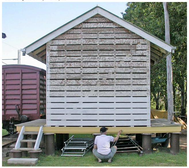
Note the location of the name board and the width of the diagonal brace, likely 1" x 3" timber inset into the vertical studs. While the exterior of the building (and outside edge of the studs, etc.) was painted white, the interior timber had either been painted a dark colour or had weathered dark. Lynn Zelmer photo, 2005.
