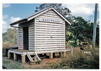
The opposite end of the Many Peaks cream shed some time prior to its removal to North Bundaberg. Note the diagonal bracing visible under the siding. The gray patch on the side appears to be the location of a power panel; the electrical conduit is visible to the left of the stump. Bundaberg Railway Historical Society photo.
