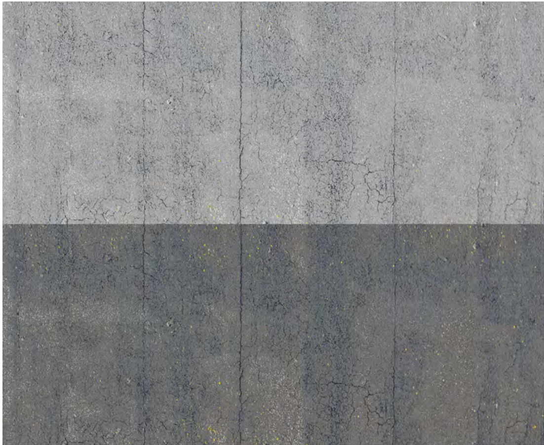
Roofing material: fold light side under, glue and trim to fit with roughly 6-8 scale inch overhang on all sides.
