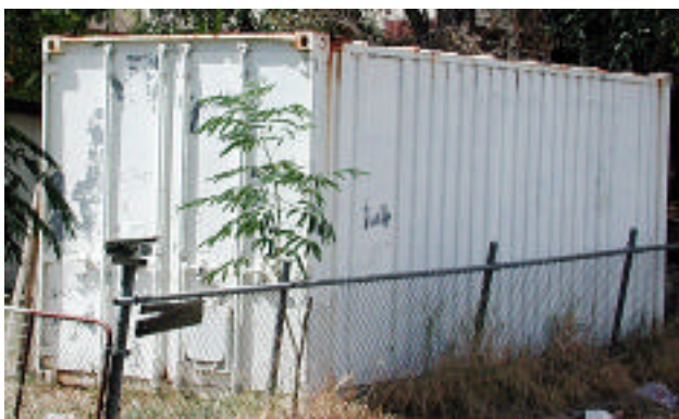
Prototype for a similar 20' container now used as a backyard shed. Note that the flat area on the side is not door width, thus the need to extend into the ribs.
