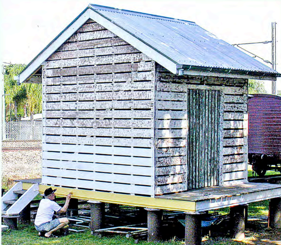
The Manypeaks cream shed while being restored at by BRHS, North Bundaberg, May 2005. The shed originally sat on squared concrete stumps with their corners chamfered and the guttering fed into a nearby water tank. Here it has a new roof and round stumps; the old paint has all been scraped down for a white undercoat and cream finish paint. Photo by Lynn Zelmer.
